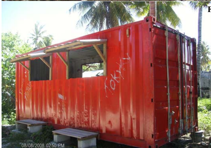
Figure 13 - New waste collection point Betio
