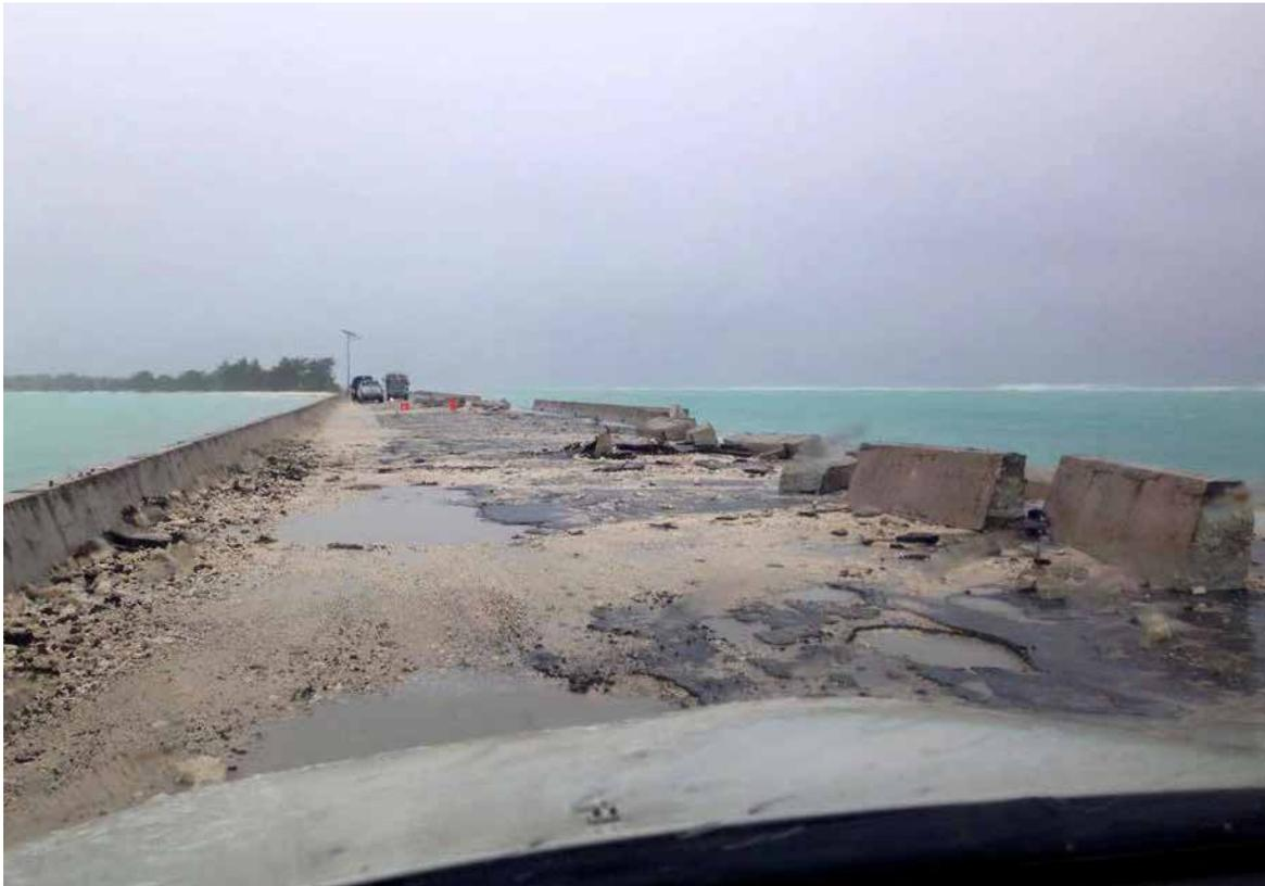
**FIGURE 9** • Damage to a causeway in South Tarawa in March 2015 caused by an intense low pressure system that later became Cyclone Pam
